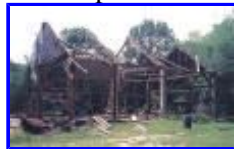
(The 30 x 40' barn being carefully dismantled on Aug. 26, 2001)
