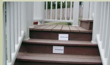
Entrance with engineered plastic decking.
