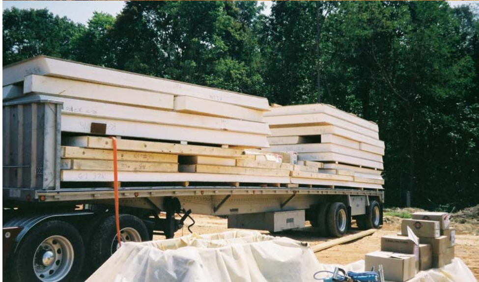
SIPs arriving at the job-site.
