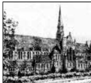
The brick church from 1888 was bombed during WWII.
