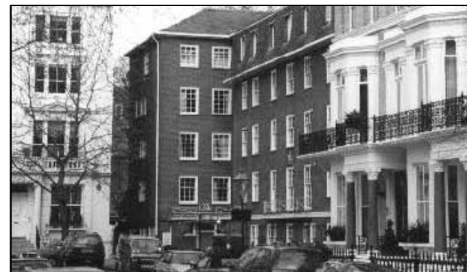
Today Vicarage Gate House stands on the old church ground.
